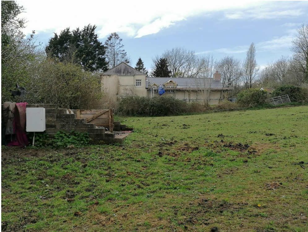
Photograph of Heronston Hall, taken from the sites entrance
